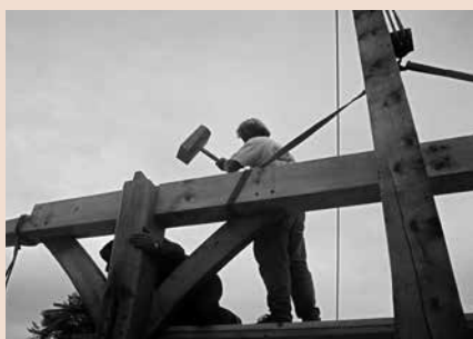
Here a section of the purlin plate has been set on the post tenons and is being "persuaded" home by Dave Bowman wielding a large wooden mallet called a persuader, beetle, or commander.
