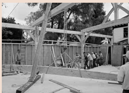
One of the big tie beams is being raised by six lodge brethren. The six-part block and tackle multiplies their force by six times. Note the pulley at the base of the gin pole that changes the direction of pull to horizontal.
