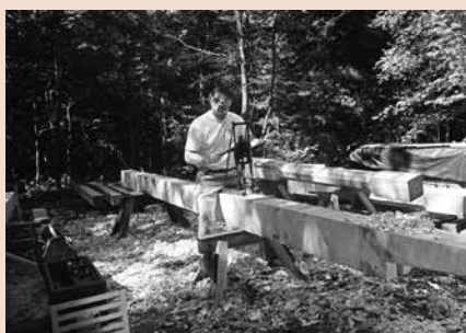
Here, Jack Sobon is cutting out mortises on a purlin plate using a 150 year old "boring machine". Note the octagonal "gunstock" posts in the background.
